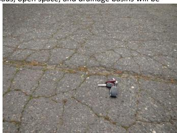
Woodfair Way – typical photo showing alligator'd pavement with grass growing in cracks. Woodfair and Rappahannock must be repaved as part of the project.
